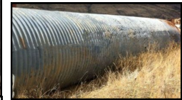
6' DIA X 20' CULVERT
